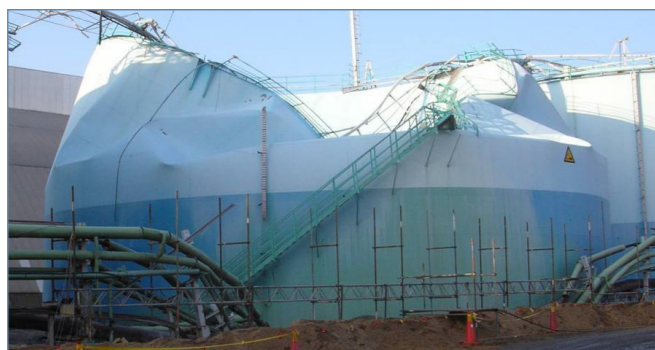
Figures 1 and 2: The damaged tank and underground pipeline (Source: Swedish Investigation Board report).
