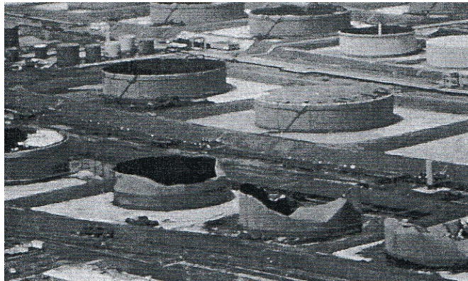
Figure 17: Petroleum Storage Tank - Hurricane Hugo (Photo Courtesy of NOAA)
